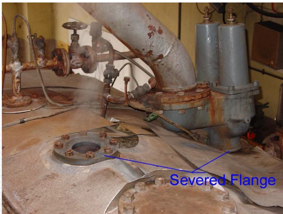
Figure 8 — Example of the effect of inadequately supported pipework
